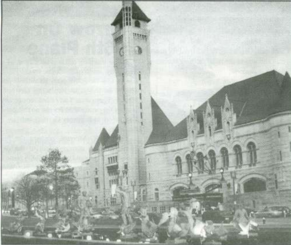
Union Station, St. Louis, a most imposing structure no longer houses trains and passengers, but is now the home of a number of restaurants and a large mall.
